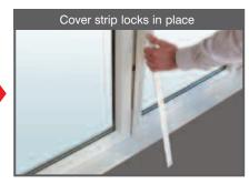
Once locked into position the Buttons are used to locate the cover strip.
