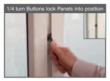
Rotating the 1/4 turn Button with an allen key secures the Panels and ensures they are the correct distance apart.
